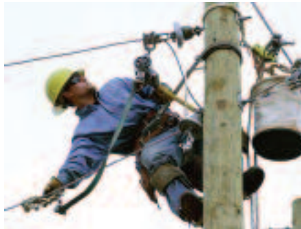
Tri-County lineman Chris Coates works to achieve the desired line tension during the sagging event. A meter reader/first-year apprentice, Coates placed 13th in the apprentice competition.
