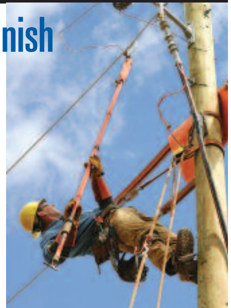
Tri-County journeyman lineman Jim Succowich uses a hot stick to energize a cut-out during the underground changeover event at the Third Annual Gaff-n-Go Rodeo and Expo April 2. The local crew finished ninth out of 20 teams entered in the linemen's competition.
